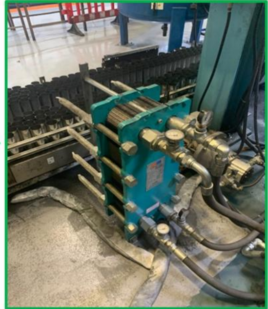
Figure 4. Transition from shell and tube heat exchanger to plate heat exchanger.
