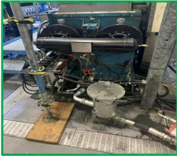
a) Renewal of pipes, fittings, and elbows
