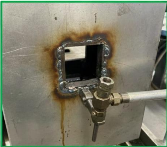
c) Sealing of "Coffin Hole" (Structural leak prevention).
