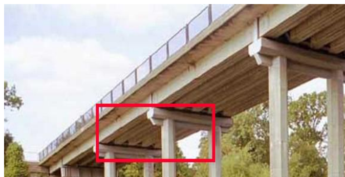
Fig. 18. Overview of the RC bridge.
