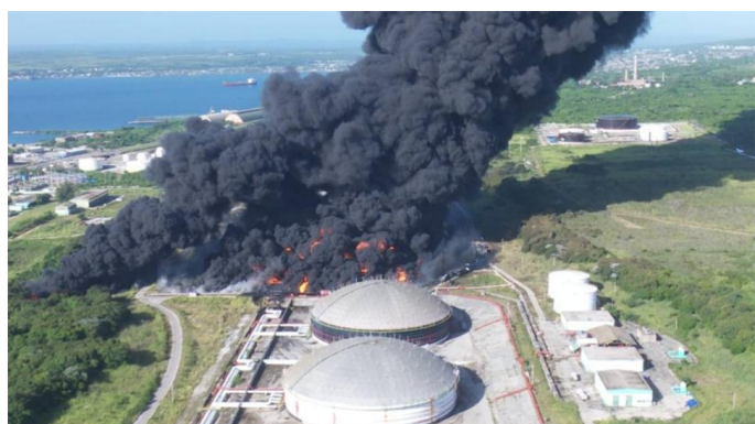
Fig. 1. A fire and explosion accident of an oil depot in the port of Matanzas Province, Cuba.
