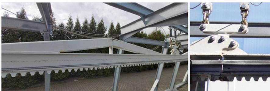
Fig. 1. View of the reinforced rail and double sling coupler built on a route intended for high-speeds [5]
