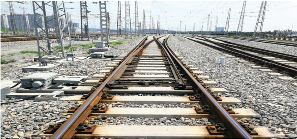
Fig. 1. Railway track switch
